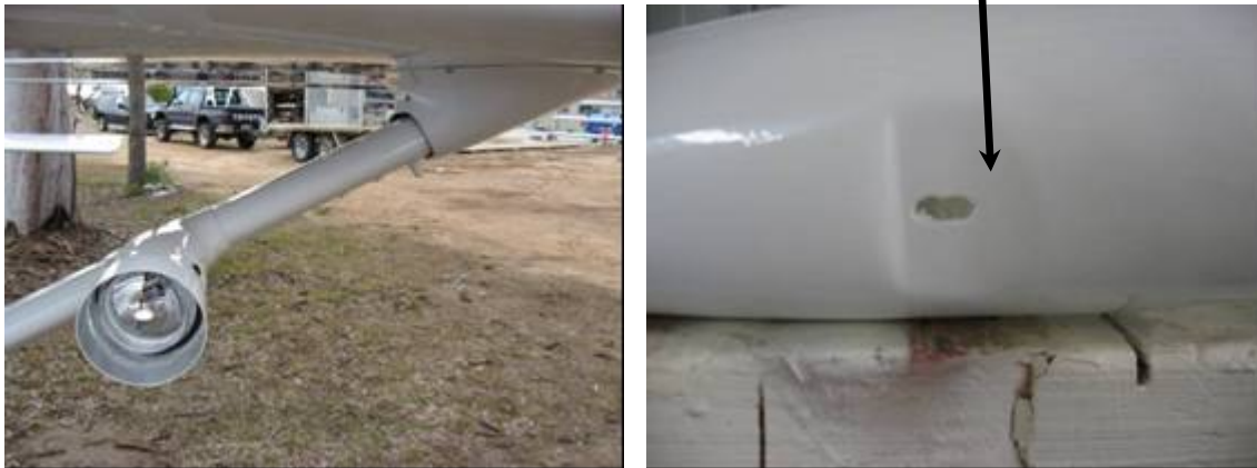
Figure 39 – Light Installed (Left) & Slotted Hole In Housing
